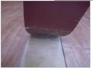
Failure – planks lifting at corners and sides. Inspection Findings - No adhesive transfer to the back of the plank. Cause – Adhesive set before plank install
