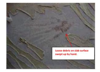
Failure – Vinyl bubbling/lifting away from slab. Inspection Findings – Bond failure between slab and adhesive bed. Cause – Adhesive could not bond to slab because the proper prep work/cleaning was not done prior to install.
