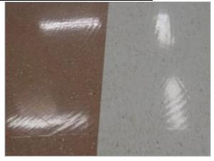
Failure – Ridges visible in flooring. Inspection Findings – Rolling floor after install did not flatten out adhesive trowel marks. Cause – Adhesive set before plank install
